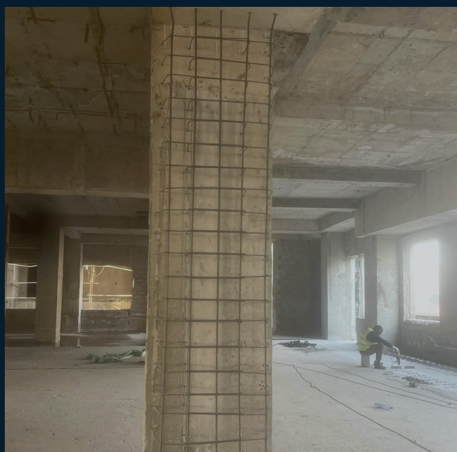
Column reinforcement / Renforcement de poteau
