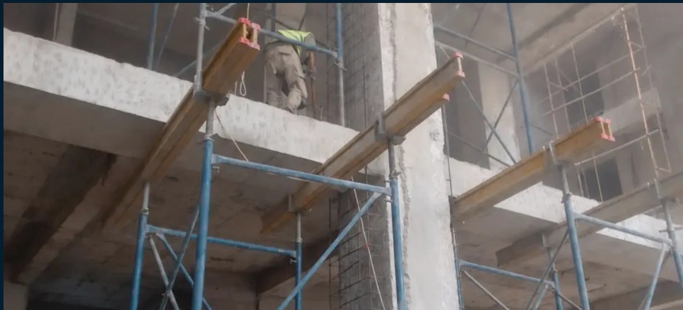
Structural retrofit / Renforcement structurel
